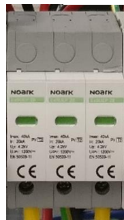
Picture 6 – Lightning arrester SPD
